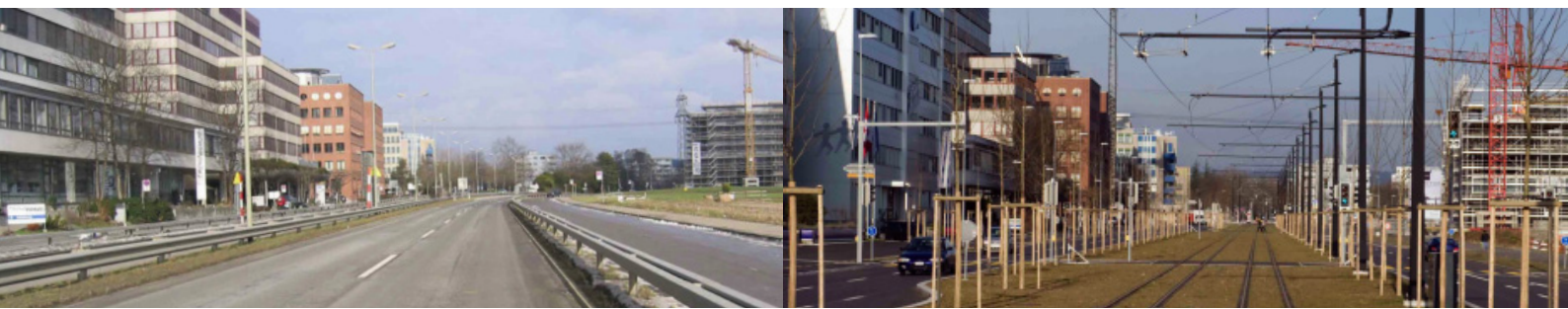
Figure 5: Glattalbahn: before and after photos (same cross-section as Figure 4. Source: VBG)
